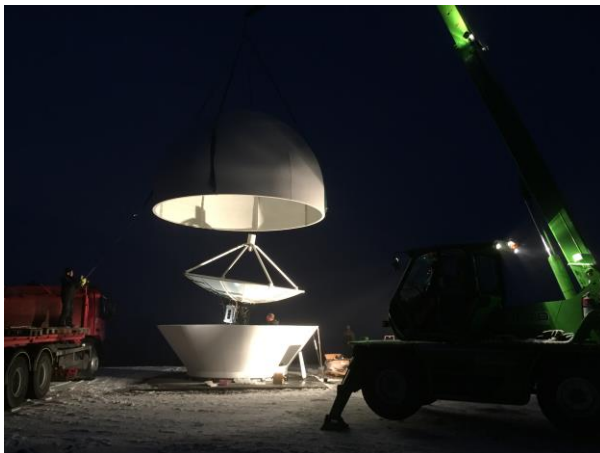
Exhibit 4: Unpacking of small antenna for SSC Infinity
